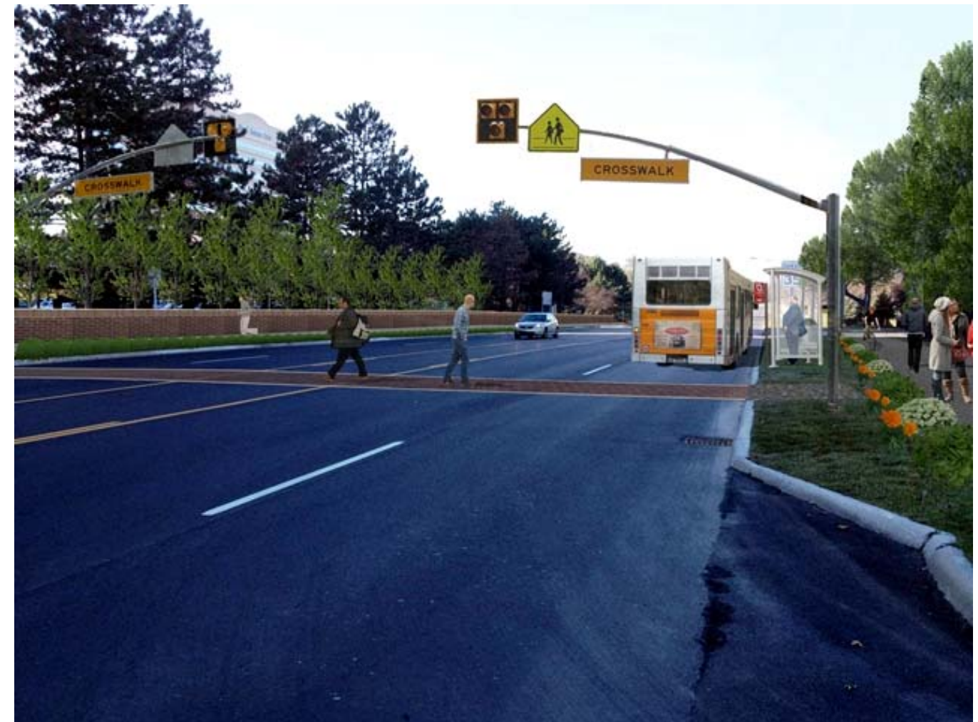
Potential mid-block pedestrian crossing showing decorative crosswalk, HAWK pedestrian signal and Southfield / SMART bus shelter with enhanced landscape plantings.
