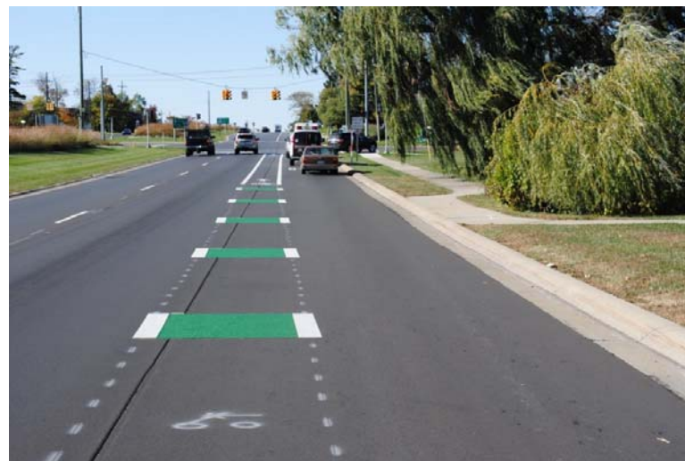
Northwestern Highway Bike Lanes: On-road bike lanes placed in 2012 by MDOT as part of an asphalt resurfacing project on Northwestern Highway (M-10) between Franklin and Inkster Roads. The bike lanes were created by restriping the existing shoulder width.
