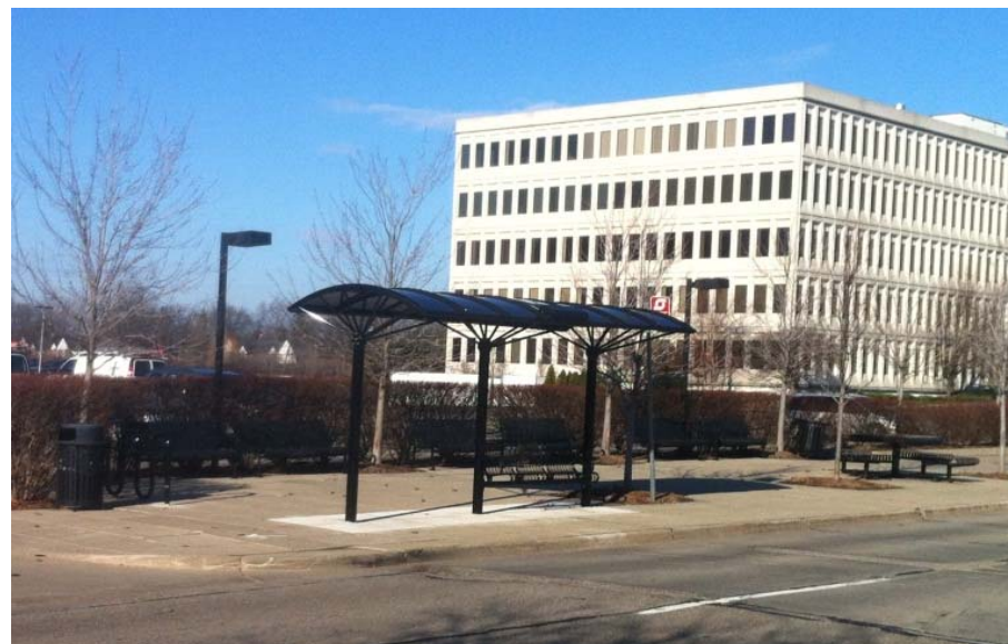
Solar Transit Stop at Southfield City Centre Plaza
