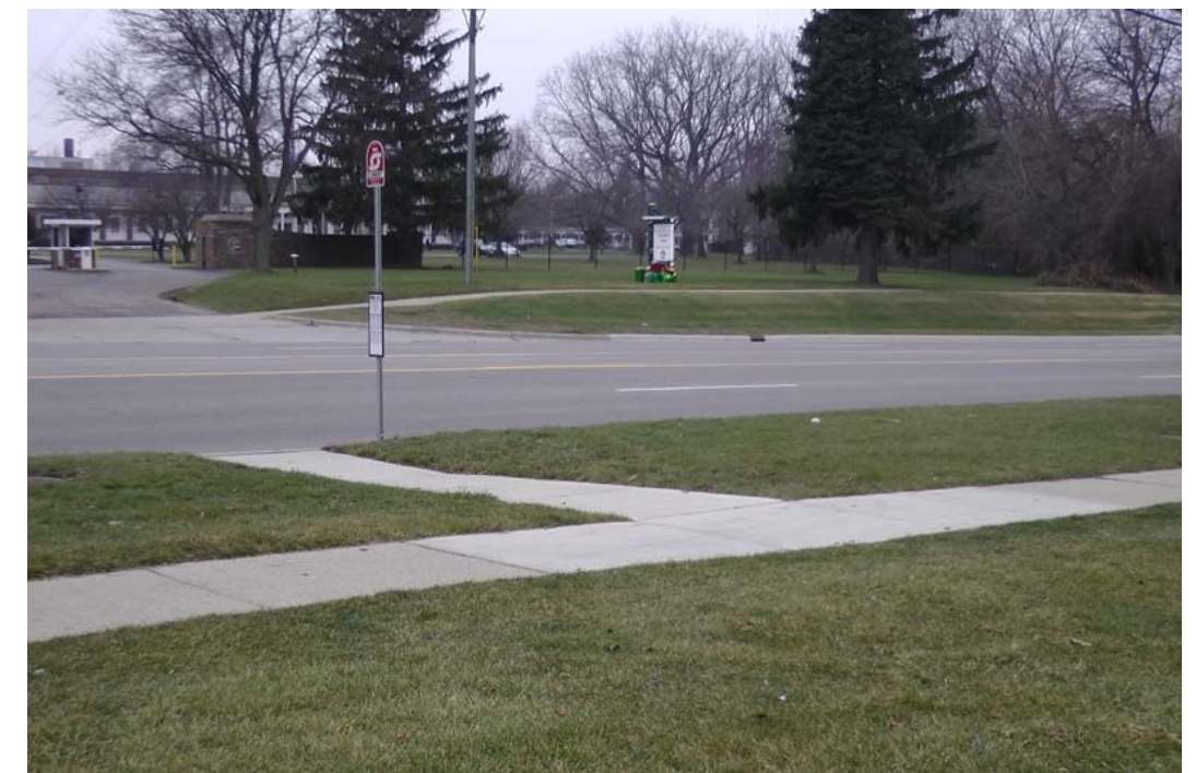
Existing SMART bus stop with ADA compliant “keywalk” (Ten Mile Road between Northwestern and LTU entrance drive)
