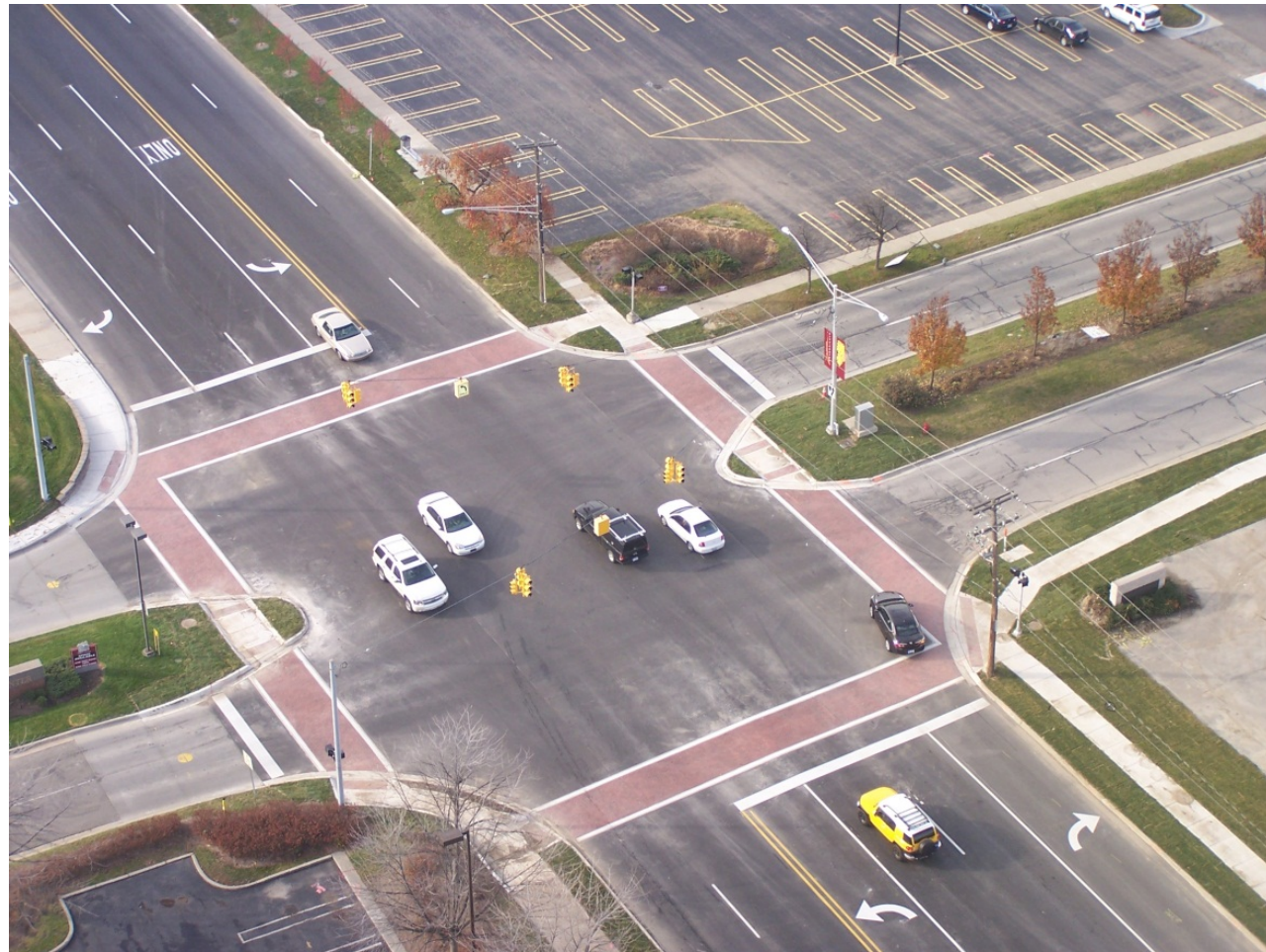
Decorative Crosswalks: Intersection of Civic Center Drive and Central Park Boulevard showing decorative crosswalks installed with resurfacing project completed in 2012.
