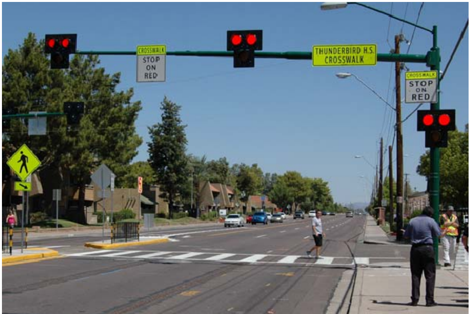
Mid-block pedestrian HAWK style signal with refuge island placed in the center left turn lane.
