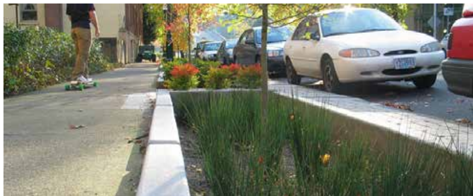
Street-side rain gardens collect stormwater runoff from streets and sidewalks, allowing more of it to percolate into the soil instead of being discharged into storm sewer system.
