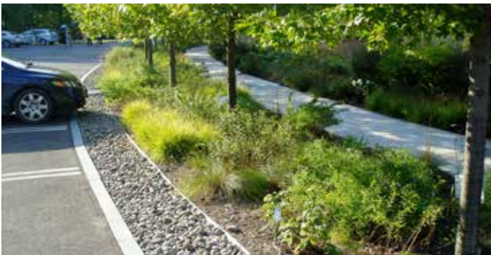
A parking lot utilizing Low Impact Design (LID) strategies, including permeable paving, a stone infiltration strip, and a bioswale.
