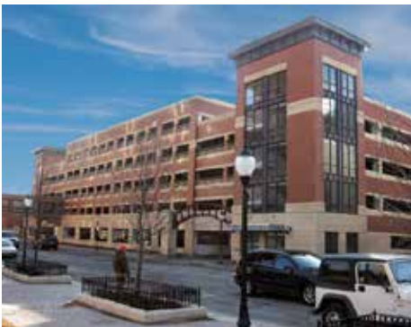
Parking garage stairwells should be designed to fit seamlessly with the rest of the parking garage's exterior.
