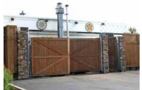
All service, equipment, and trash enclosures shall be screened on all sides, including an appropriately styled gate.
