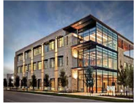
Single use building oriented toward the street.
