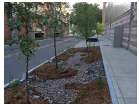
Bioretention can be used as a buffer from pedestrians and roadways while providing environmental benefits.
