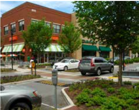
Bioretention can be used as a buffer from pedestrians and roadways while providing environmental benefits.
