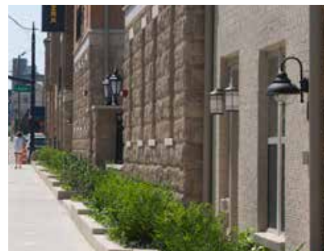
Wall-mounted lighting should blend in with the building frontage.
