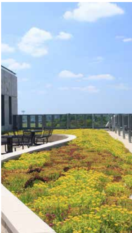
Green roofs reduce stormwater runoff, energy use, and the heat island effect.
