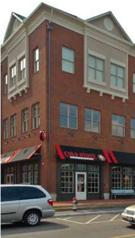
EIFS should only be used on the 3rd story and above of any building within the development.
