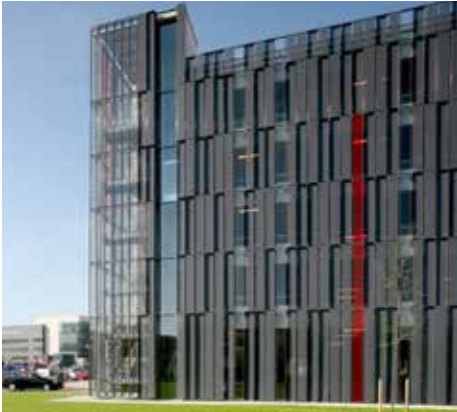
Structured parking lots can be screened with high quality materials.
