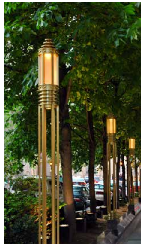
Selecting consistent lighting structures helps reinforce a brand or identity throughout the development.
