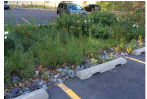
Rain gardens within parking areas provide landscaping while also absorbing and filtering stormwater runoff.
