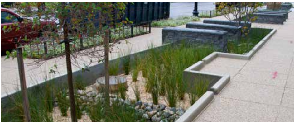
Rain gardens and bioswales should be designed per current best practices. These basins are typically designed for water to percolate into the soil over a 24-48 hour period, thereby limiting long periods of standing water and attraction to mosquitoes.
