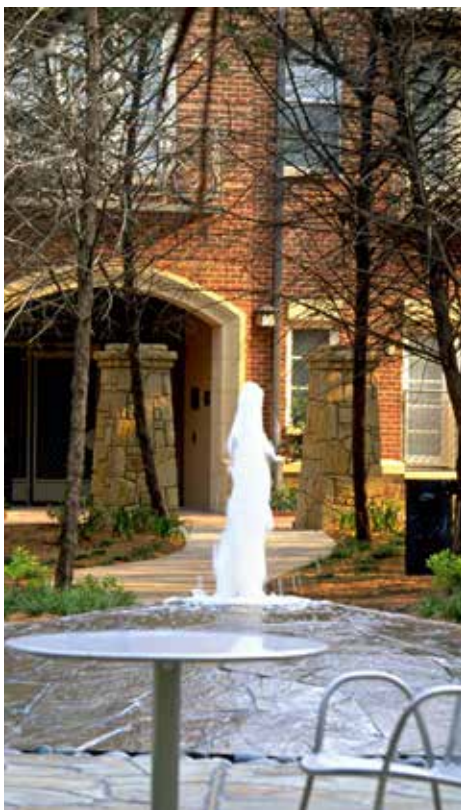
Carriage way entries provide access to public and private courtyards and plazas.
