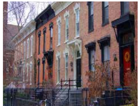
Townhomes fronting the street will help the Central Park District retain a walkable, community feel.
