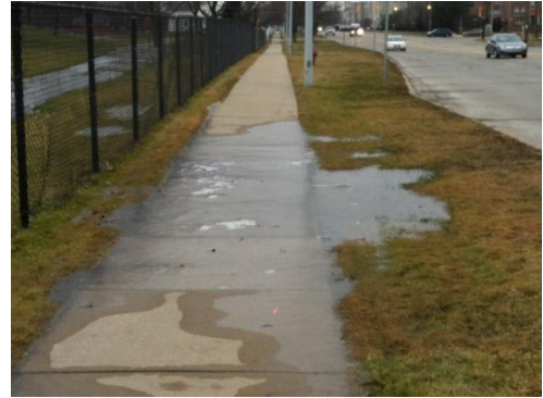
Lack of drainage results in wet, slippery pathways that are often not passable.
