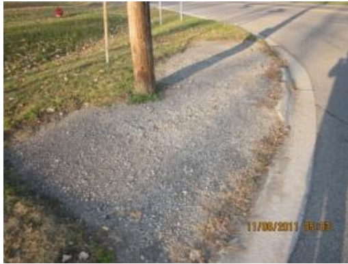
This pedestrian pad is constructed of inadequate materials, creating safety and maintenance issues.
