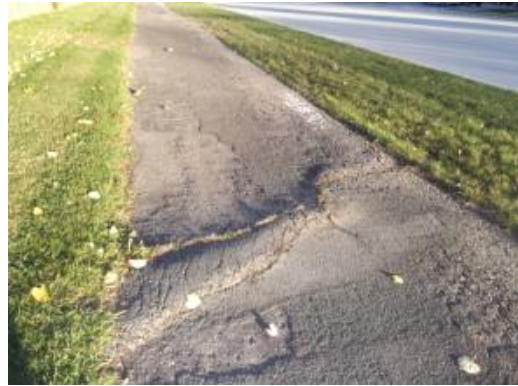
Settling and tree routes often interfere with the safety of a non-motorized path.
