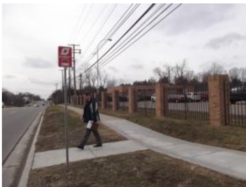
Properly installed keywalks enable safe bus access.
