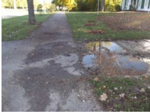
Non-motorized paths should not drain into existing driveways, roadways, or yards.
