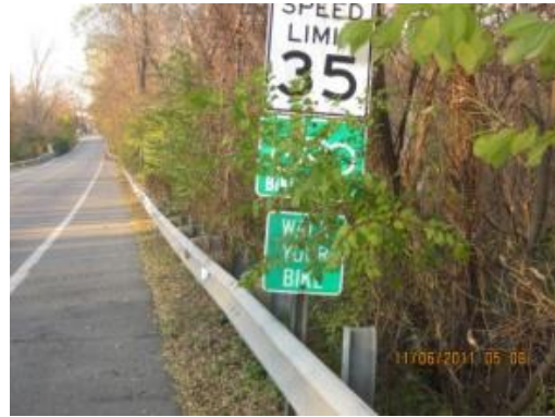
While not directly affecting the path, overgrown landscape can interfere with usage by reducing wayfinding sign visibility.
