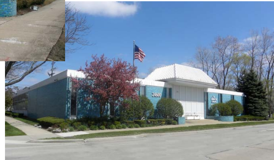
The Albrecht Companies (1964) (Note colorful glazed brick that was popular in 1960s construction.)
