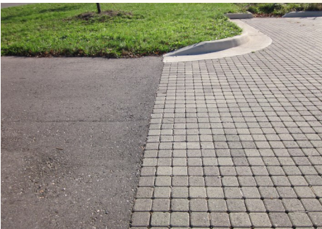
Pervious Pavers at Carpenter Lake
