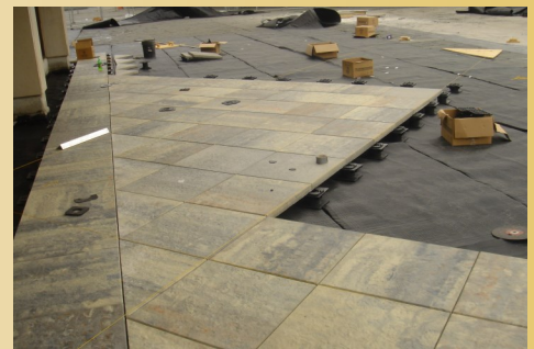
Precast concrete paver on Terra-Adjust Pedestal System at City Hall
