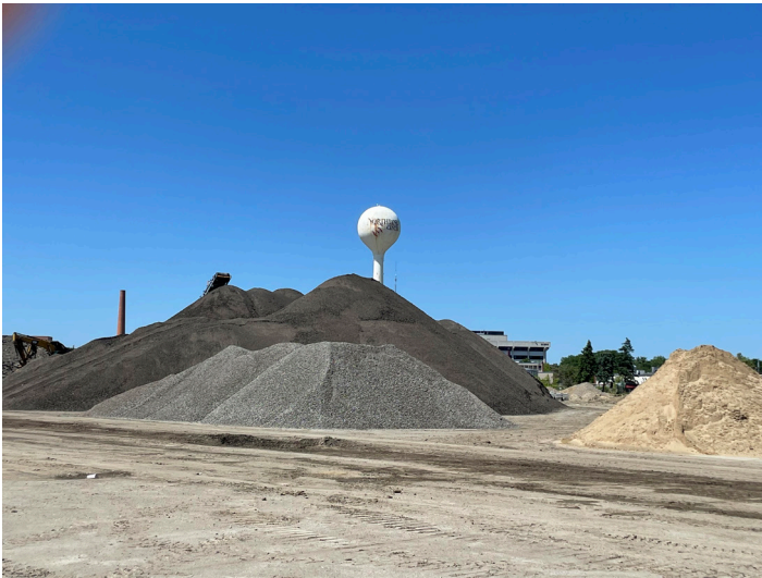
At one time Northland Center had 10,000 surface parking spaces. Contour Companies has lifted the blacktop and milled it for reuse. Milled blacktop is in piles in photo above. Steel, aluminum, concrete and bricks are also being recycled.
