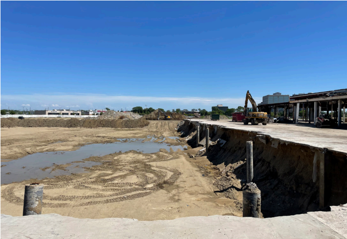
The former JC Penney's store has been demolished. Stored dirt on the site is now being used to fill in what was the store's basement. The original 1954 Northland structures are being save for new uses.
