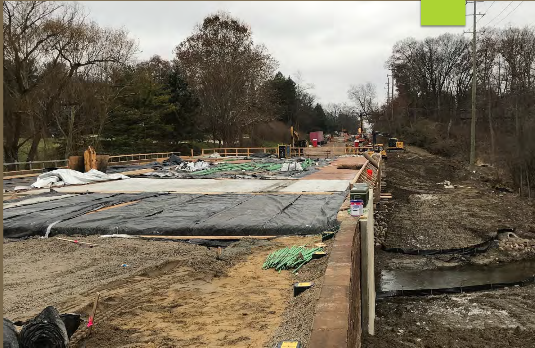
Nine Mile/Lahser Road bridge replacement under construction
