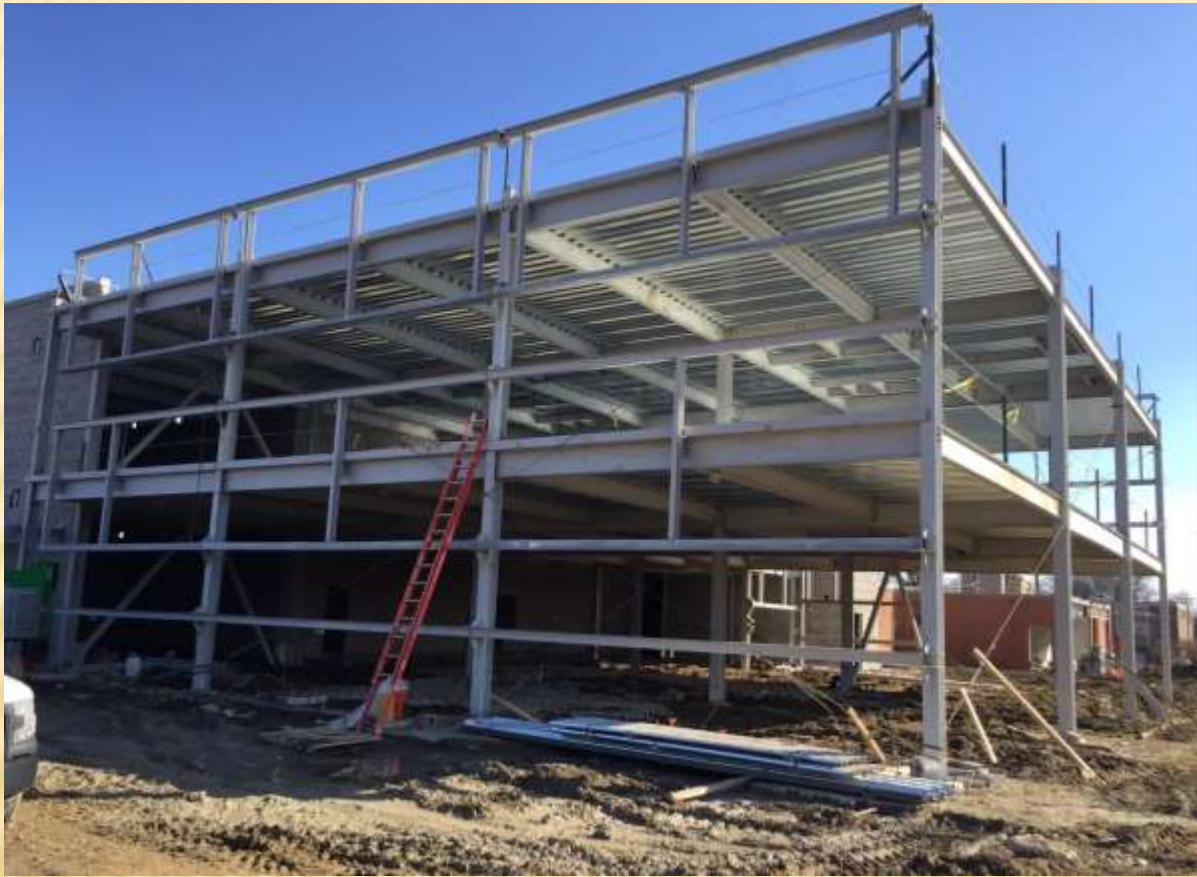
New Yeshiva Beth Yehudah under construction.
