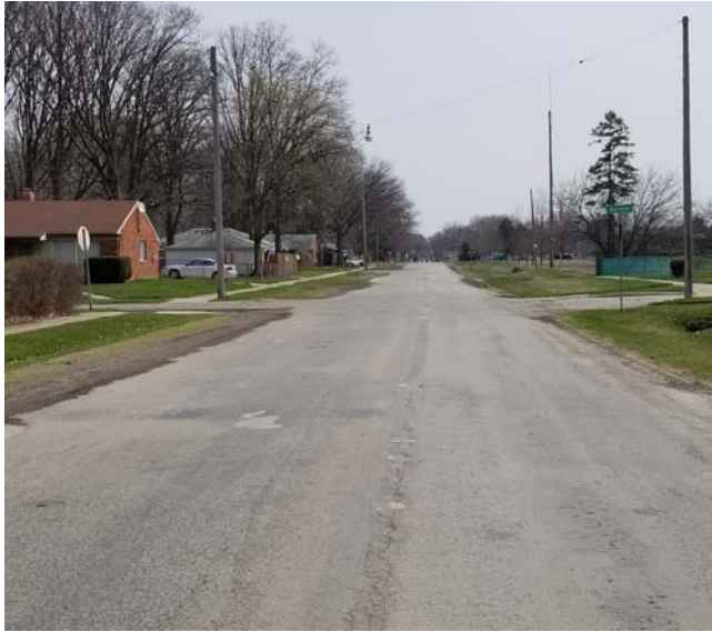
Catalpa Street (Full Asphalt Reconstruction and Open Cut Water Main)
