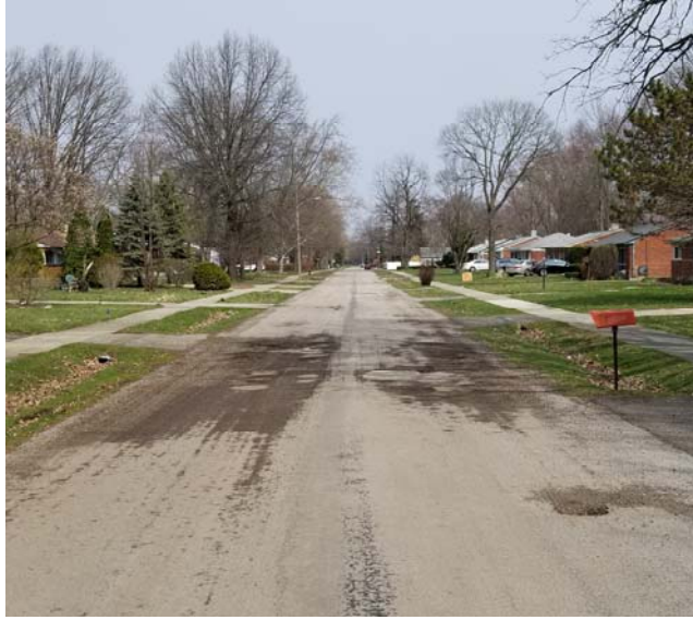
San Rosa, Wiltshire, Aberdeen, Selkirk, Fairfax, Marshall, Brentwood Canterbury Gardens (Asphalt Pulverization; Open Cut Water Main Installation on Wiltshire, Aberdeen, Selkirk and a Portion of Everett)
